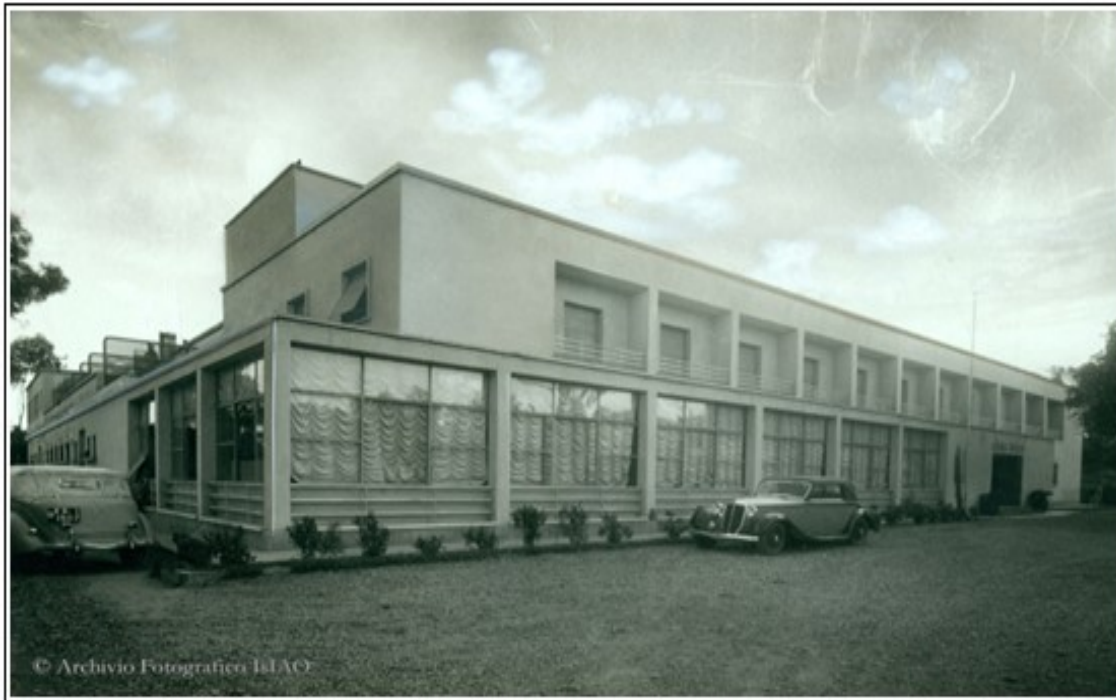
Figure 4 Selam Hotel building
