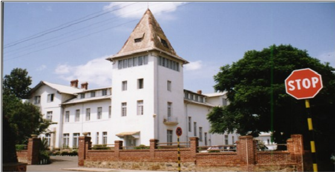
Figure 5 Hamasien Hotel building
